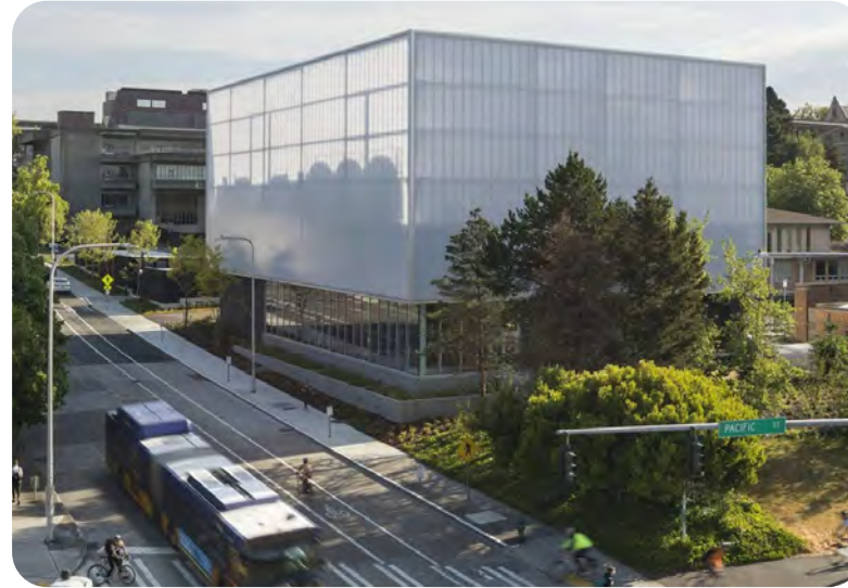
University of Washington West Campus Utility Plant (WCUP)
